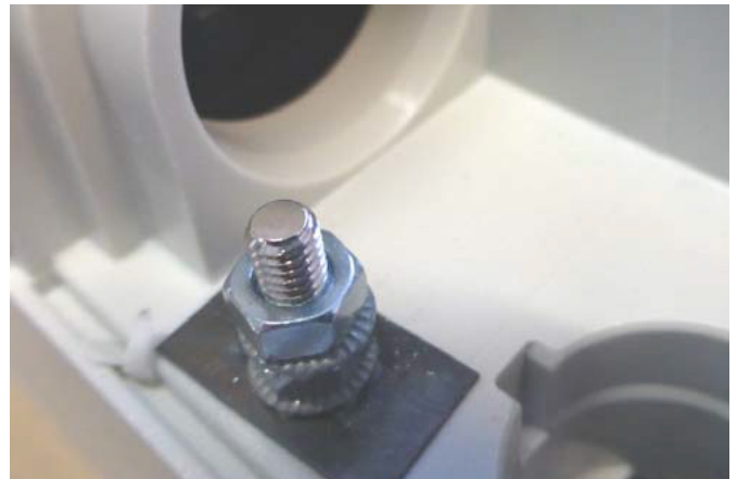
Protective earth, metal pin
