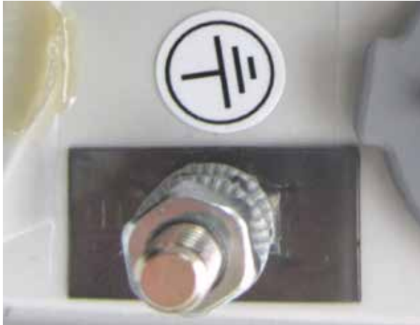
Fig. 16: Metal pin (bolt) to connect devices to PE
